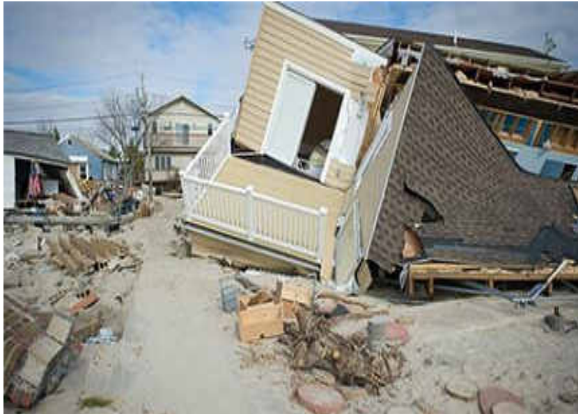
Houses damaged after an earthquake of magnitude 6.5 struck the coastal Bangkok
