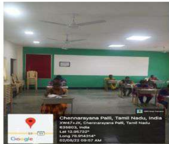
LED Lights in Smart Class (Room No. 103)
